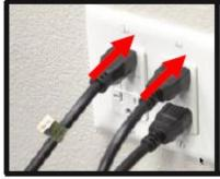
Plug in the fountain lobby electrical cords from the electrical outlet that includes the fountain dispenser and carbonator pump, turn co2 supply on.
