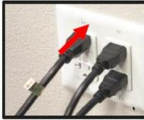
Plug the electrical cord for carbonator pump from the electrical outlet.
