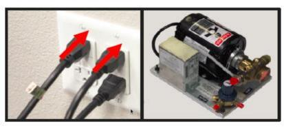
Plug in the fountain lobby electrical cords from the electrical outlet that includes the fountain dispenser and carbonator pump, turn co2 supply on.
